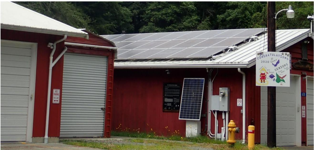
The fire hall's solar-electric system provides a large portion of the facility's electricity and also backs up critical loads during utility outages
